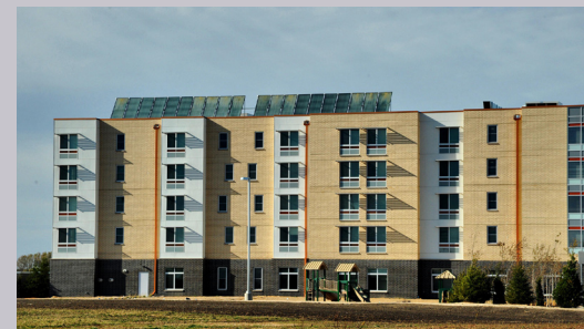
Country Club Hills Wellness Center provides permanent supportive housing for 20 families and 57 individuals via South suburban PADS. While not visible as the roof mounted Solar Thermal is, the facility is heated and cooled via a geothermal system. Copyright: Alberts Photographic
