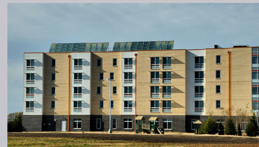
Country Club Hills Wellness Center provides permanent supportive housing for 20 families and 57 individuals via South suburban PADS. While not visible as the roof mounted Solar Thermal is, the facility is heated and cooled via a geothermal system. Copyright: Alberts Photographic
